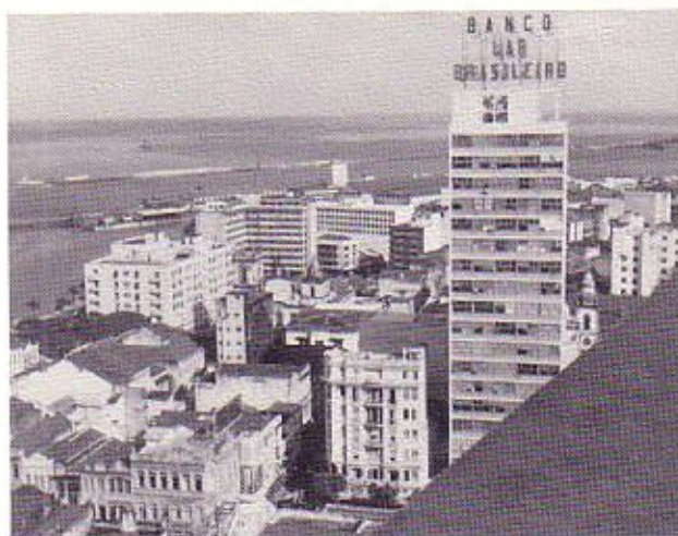
A view looking north.
