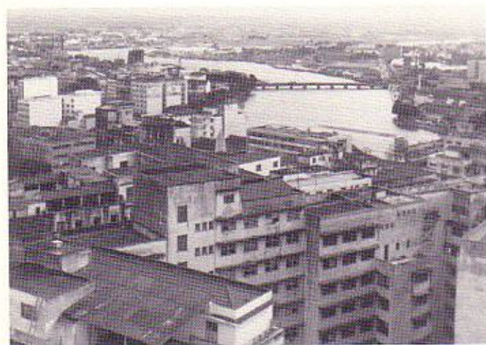
A view of the town looking south.
